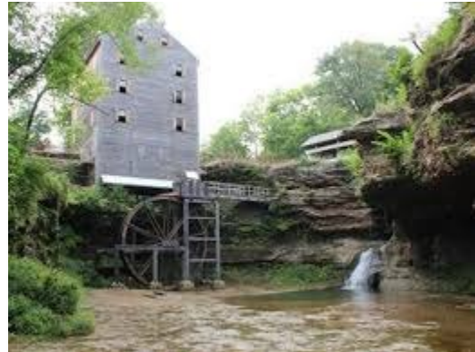
Rock Mill – Fairfield County Park District
